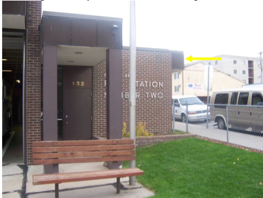
Figure 8: Campus Town Antenna Mounting Location
